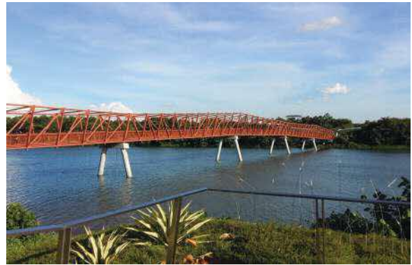
The iconic red bridge across Sungei Serangoon, 2017. Courtesy of the National Heritage Board.
