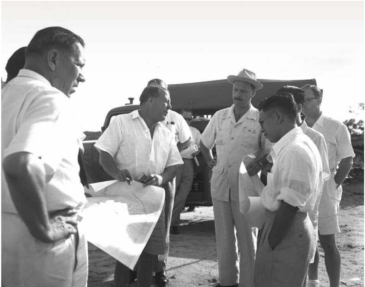
Minister for Communications and Works Francis Thomas initiates works for the construction of a dam at Ulu Bedok to alleviate floods at 9 th mile Changi Road, 1955. Ministry of Information and the Arts Collection, courtesy of the National Archives of Singapore.
