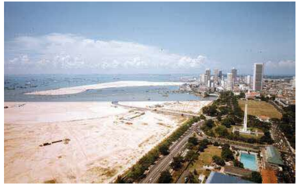
Reclamation works at Marina Bay, 1977. © Urban Redevelopment Authority. All rights reserved.
